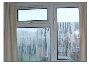
Condensation typically forms on non-absorbent surfaces such as glass, pipework or impervious painted surfaces and whilst that condensate might not damage the material on which it occurs, if there is sufficient deposit it will run and drip on to materials where it may cause damage.
